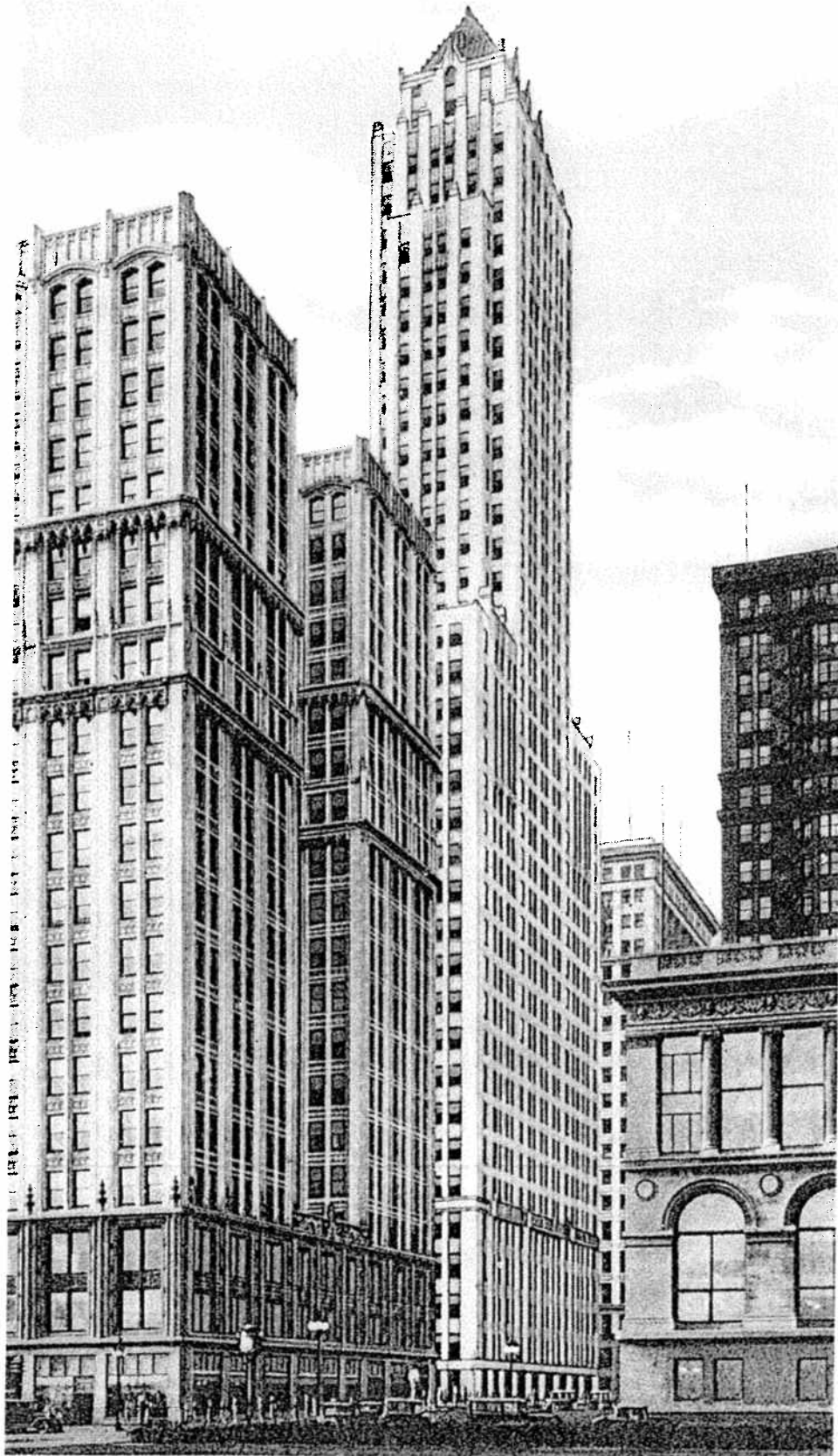
A postcard view of the Pittsfield Building, circa 1927. The building is an excellent example of a 1920s skyscraper combining both Gothic and Art Deco detailing.
